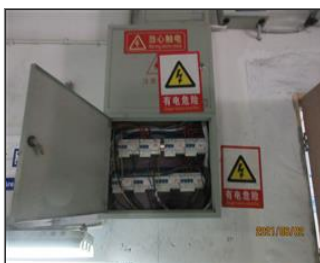
Photo of non-conformity NC 7.13 No inner cover.JPG
