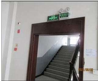
Photo of fire safety equipment 2. Emergency Light. Safety Exit Sign. Fire alarm.JPG
